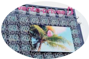
headquarters "Vente-Privée" (Paris 2015) concrete molding, RAIGI formulation
